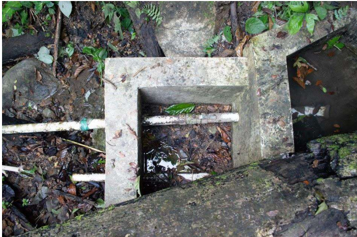
Figure A-5. Existing Quebrada Platano Big Tank Intake
